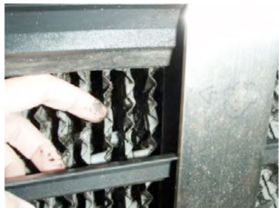
After Vulcan was installed for 5 months: the scale can be removed easily with a finger.
