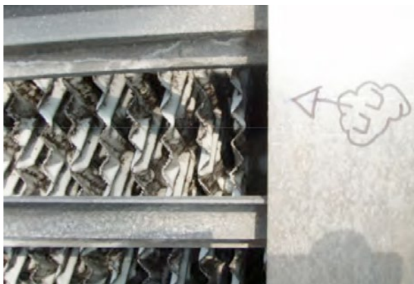
Before Vulcan was installed: the outside of the cooling tower.
