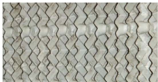
After Vulcan was installed for 5 months: the scale has been reduced.
