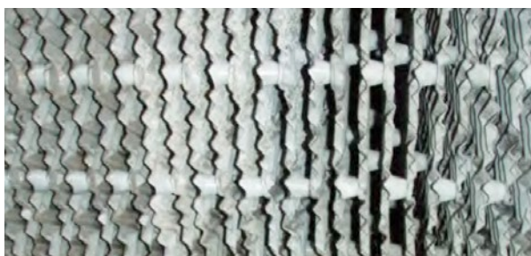
Before Vulcan was installed: the inside of the cooling tower.
