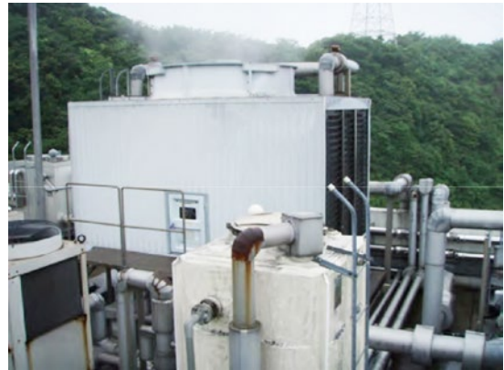
The cooling tower roof of medicine factory
