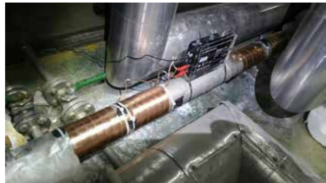
Vulcan S25 installed at Toray Industries
