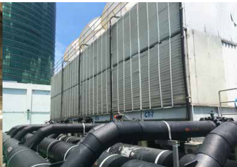
7 cooling towers were treated with Vulcan.
