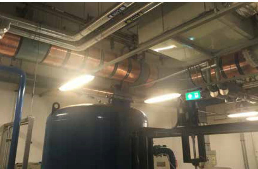
Vulcan S250 and X-Pro 1 were installed on the main return pipes of the condenser.
